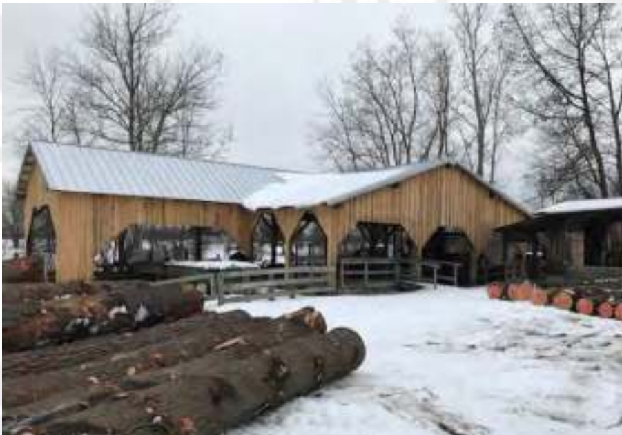
A major improvement on the Crossroads Village Sawmill was also completed after a roof was installed to help protect the equipment from the elements. All the lumber used to construct the Sawmill structure came from Park land and was processed at the sawmill.
