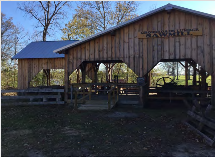
Sawmill open enclosure building
