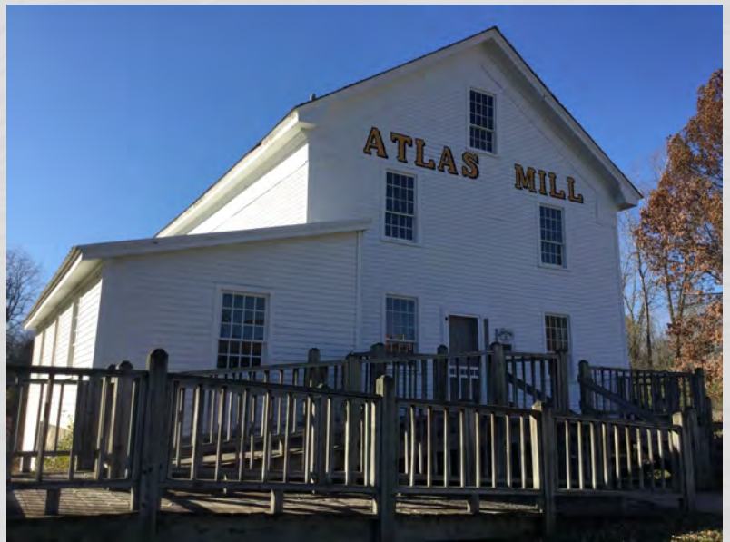
Painted and restored Atlas Grist Mill
