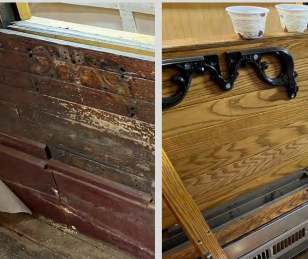
Car #306 interior wood walls restoration Left: Before Right: After
