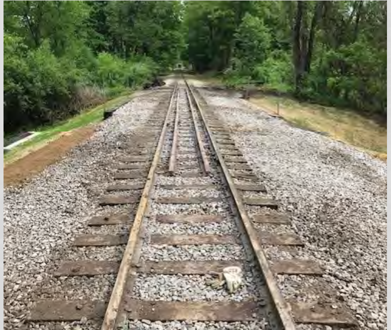
New railroad ties on the main line
