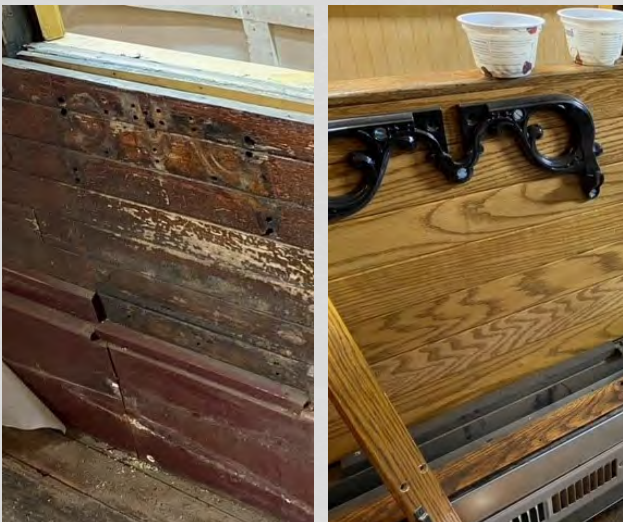
Car #306 interior wood walls restoration Left: Before Right: After
