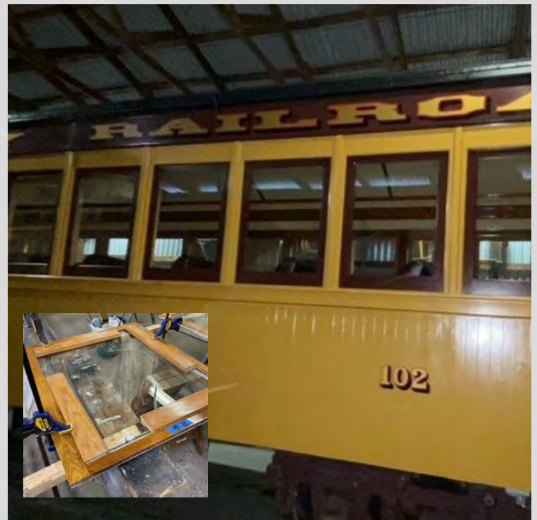
Car #102 freshly painted with new windows installed Inset: Restoring and rebuilding windows for train car restoration
